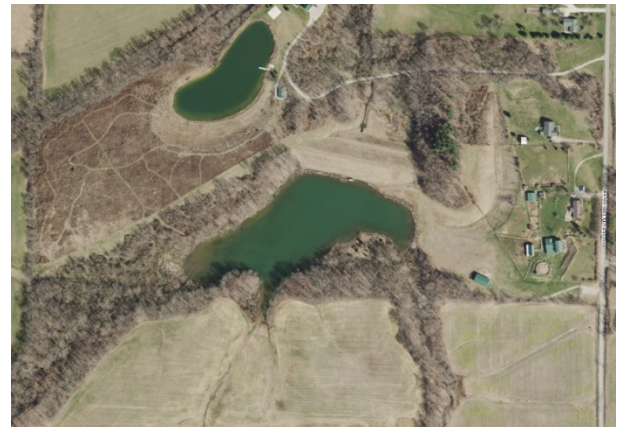
2018 Aerial Photo of Dam 4
