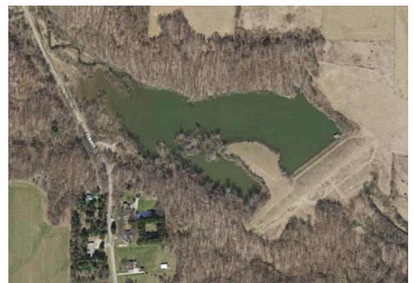
2018 Aerial Photo of Dam 9
